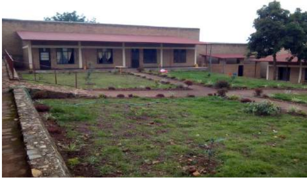
Newly constructed classrooms and compound
